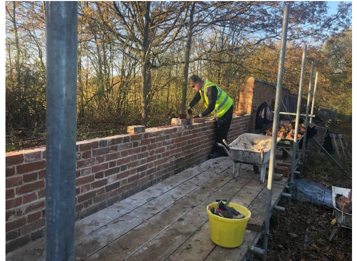
Photographs of bricklayer John Shelley on 25 th November 2021, slaking lime on the left and rebuilding a collapsed section of wall on the right
