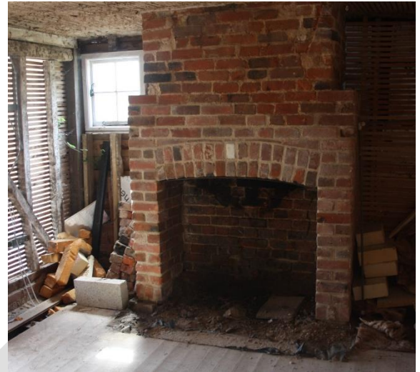
Interior showing the recently restored fireplace and new laths awaiting lime plaster. 10 th of August 2021
