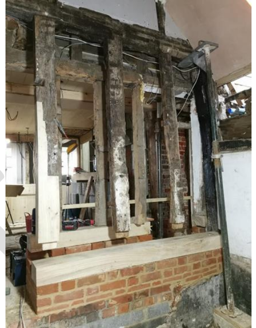
Timber-frame repairs at the Ferry Boat Inn, North Fambridge in January 2020
