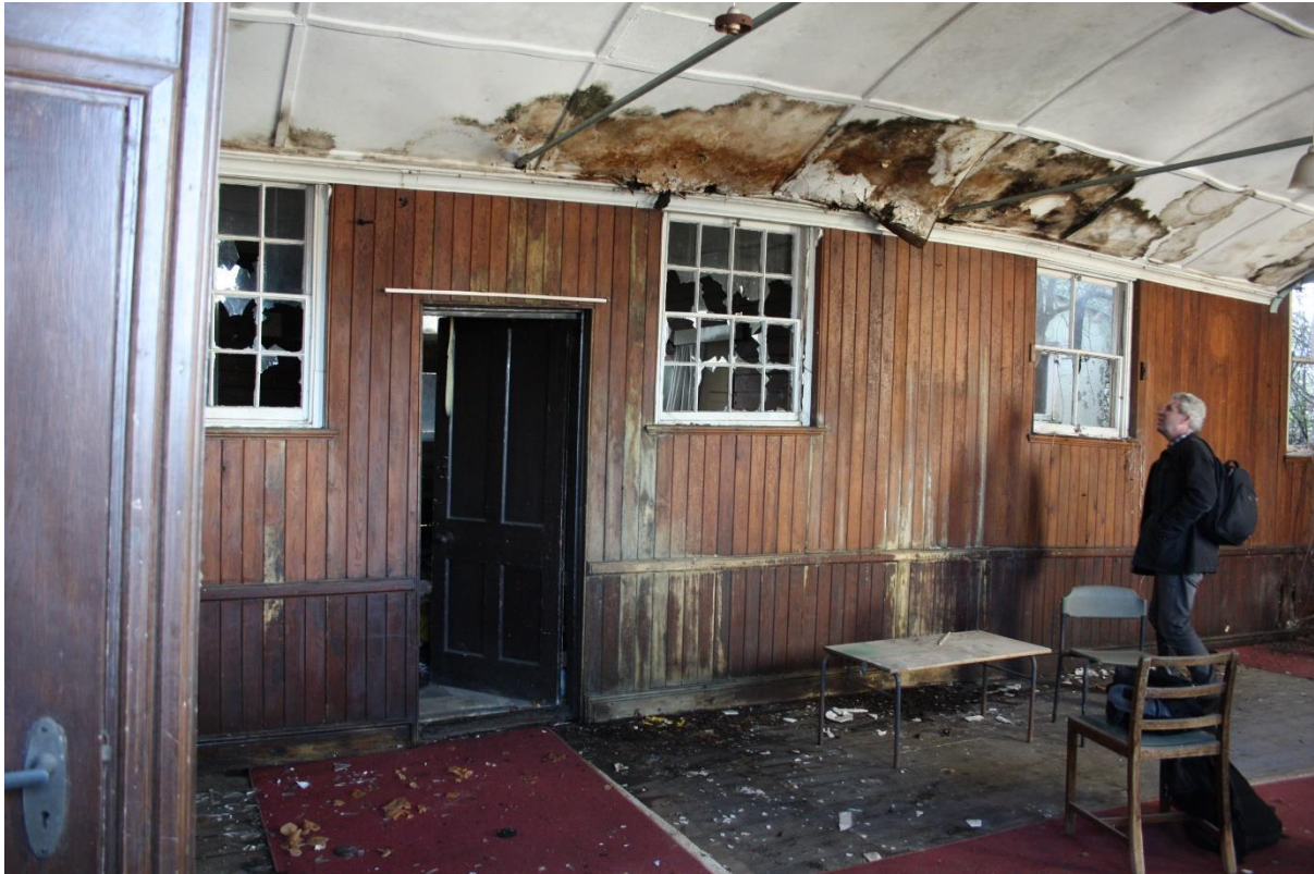
The leaking roof valley of the Heybridge Basin URC Chapel being inspected by structural engineer Ed Morton on behalf of SAVE Britain's Heritage, 5 th of February 2020
