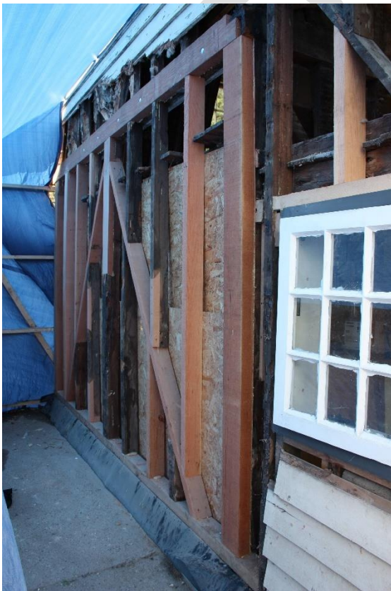
The gable end of No. 3 Black Lion Cottages undergoing repair
