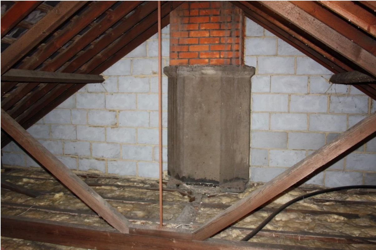
Fig. 12 - A photograph of the inside the attic of No. 155 showing an original concrete chimney
