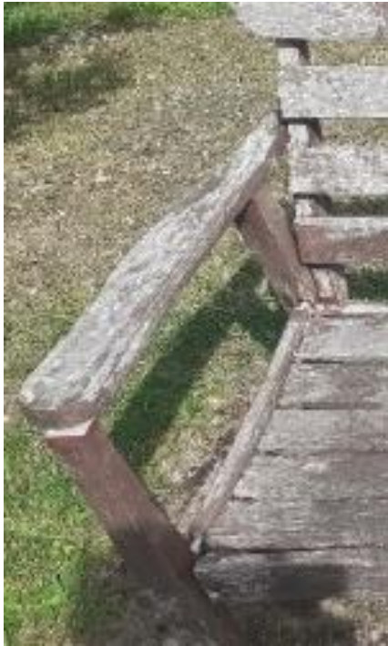
2b. cracking of wood and loose joints within the assembly of the bench.
