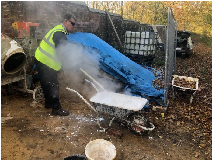
Photographs of bricklayer John Shelley on 25 th November 2021, slaking lime on the left and rebuilding a collapsed section of wall on the right
