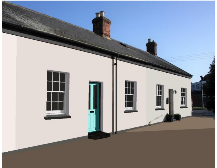
A mock-up showing how Nos 127 and 126 could be refurbished with sash windows, four-panel doors, and a resin-bonded-shingle surface to the lane.
