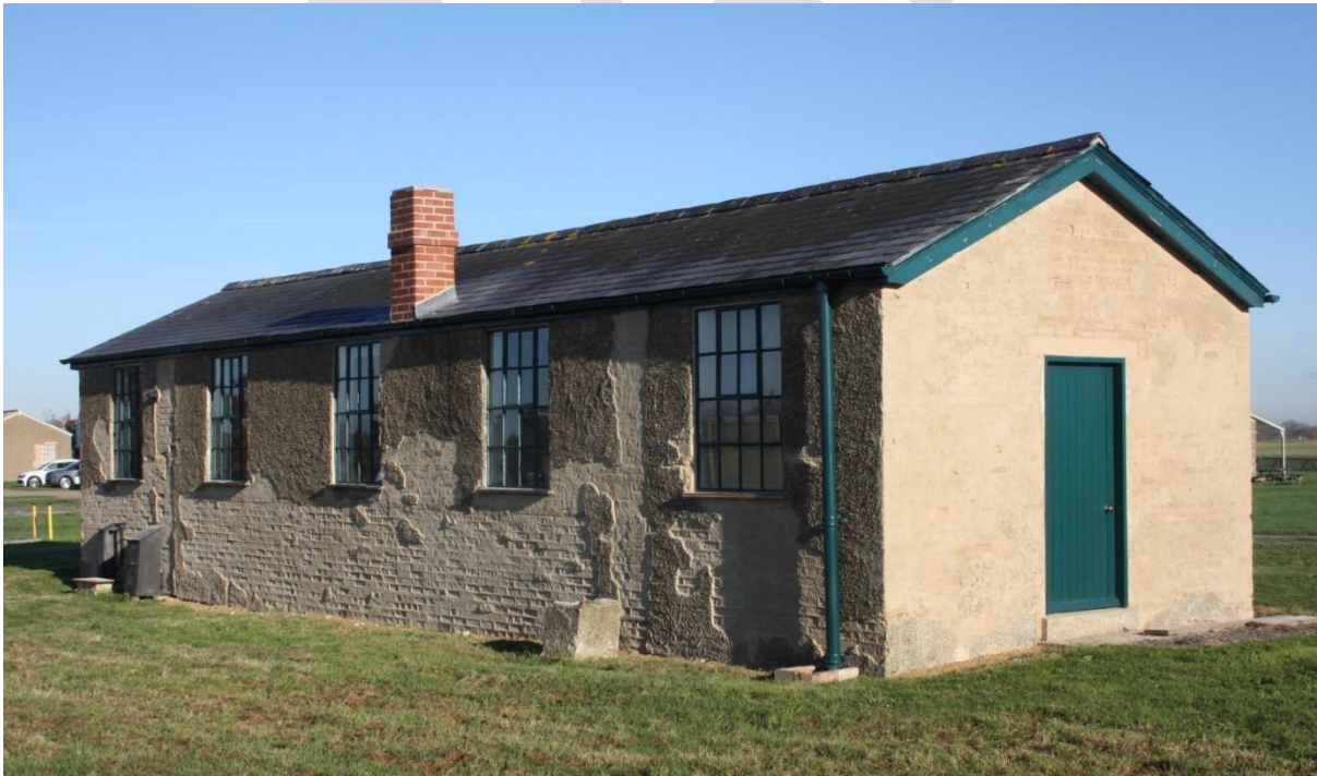
Building 30 at Stow Maries Aerodrome in November 2021. The building has been repaired in stages over the past decade, with grant support from Leader and Historic England, and is now used as offices for the trust which manages the site. The application of a protective lime-based slurry coat in October 2021 represented the final stage in the building's refurbishment and it can now be removed from the register.
